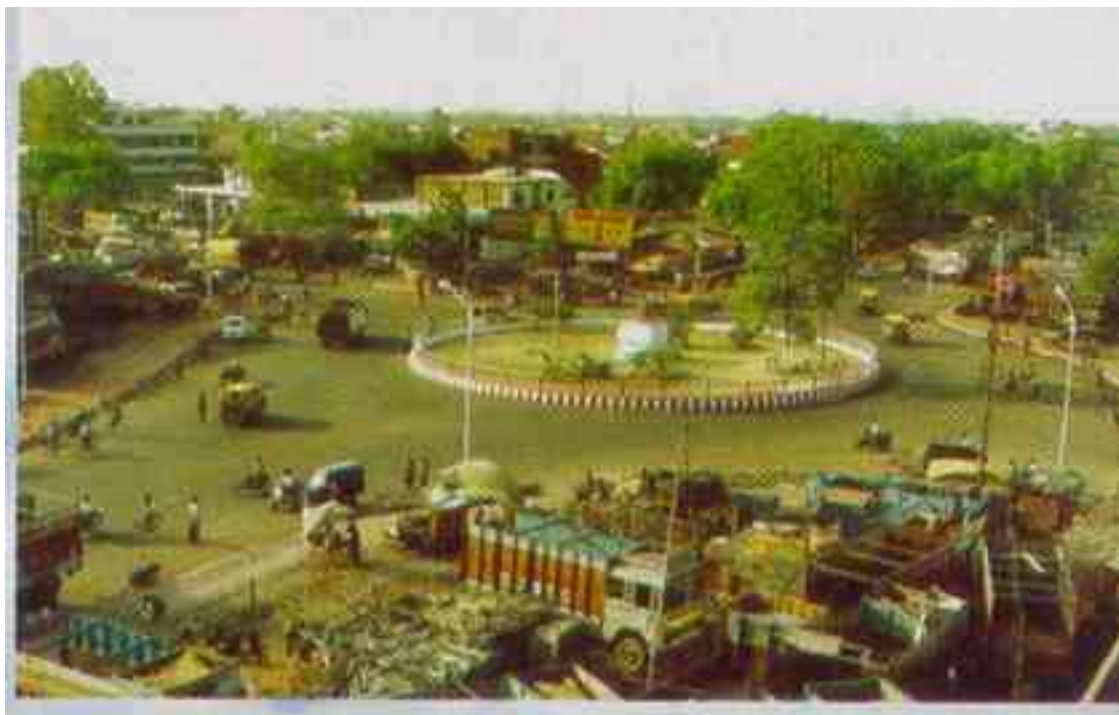
Traffic islands constructed/improved at several places for better traffic flow
