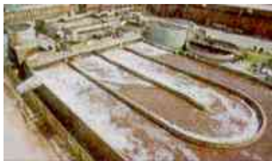
Effluent Treatment Plant of Pharmaceutical Industries
