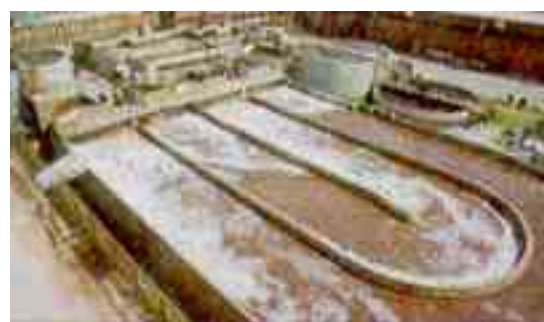
Effluent Treatment Plant of Pharmaceutical Industries
