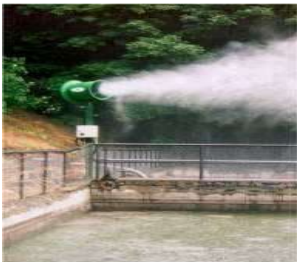
Figure 4. A typical atomizer installation for odour control
